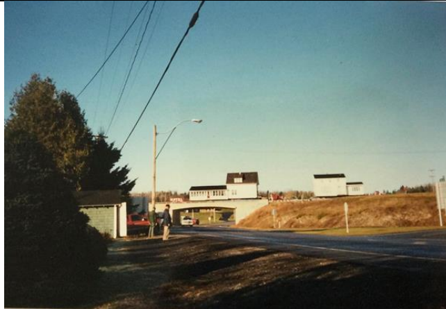
The Burke home on the final leg of its journey to its new location on Fort Road.
