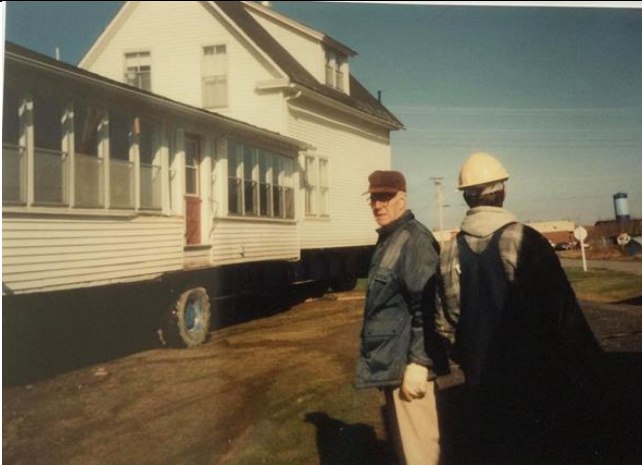
Leo Burke watching as his flood ravaged home is taken for relocation.
